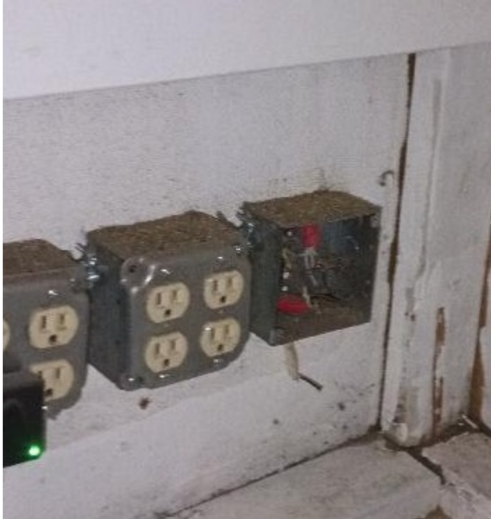
Uncovered wall box underneath of POS Counter
