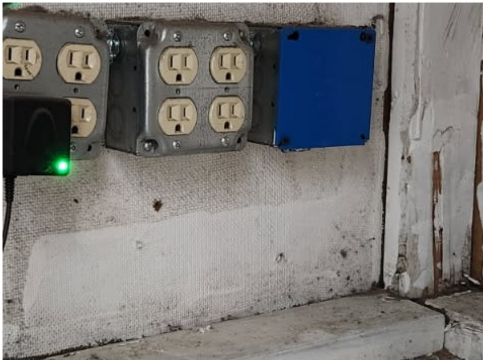
Fixed It now Wall box underneath of POS Counter is covered
