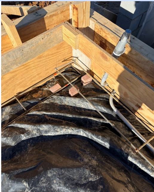
Pool house foundation rebar
