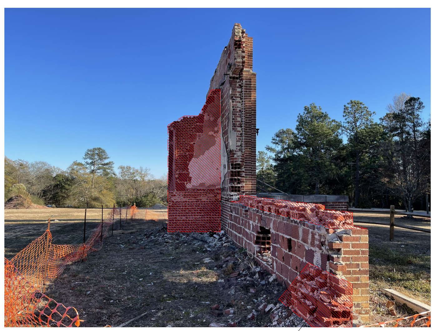
DEMO PORTION OF MASONRY
