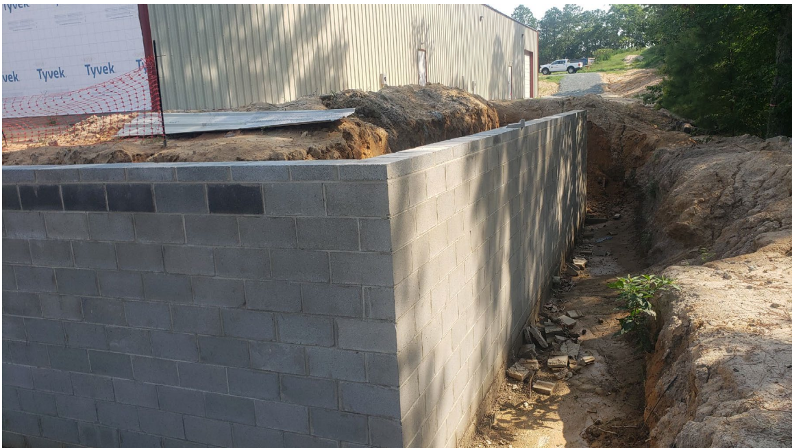
Examples of retaining wall during TE&D inspection
