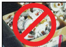
INCORRECT (Protective caps not in place)
