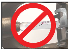
INCORRECT (bulb cracked, fluid missing)
