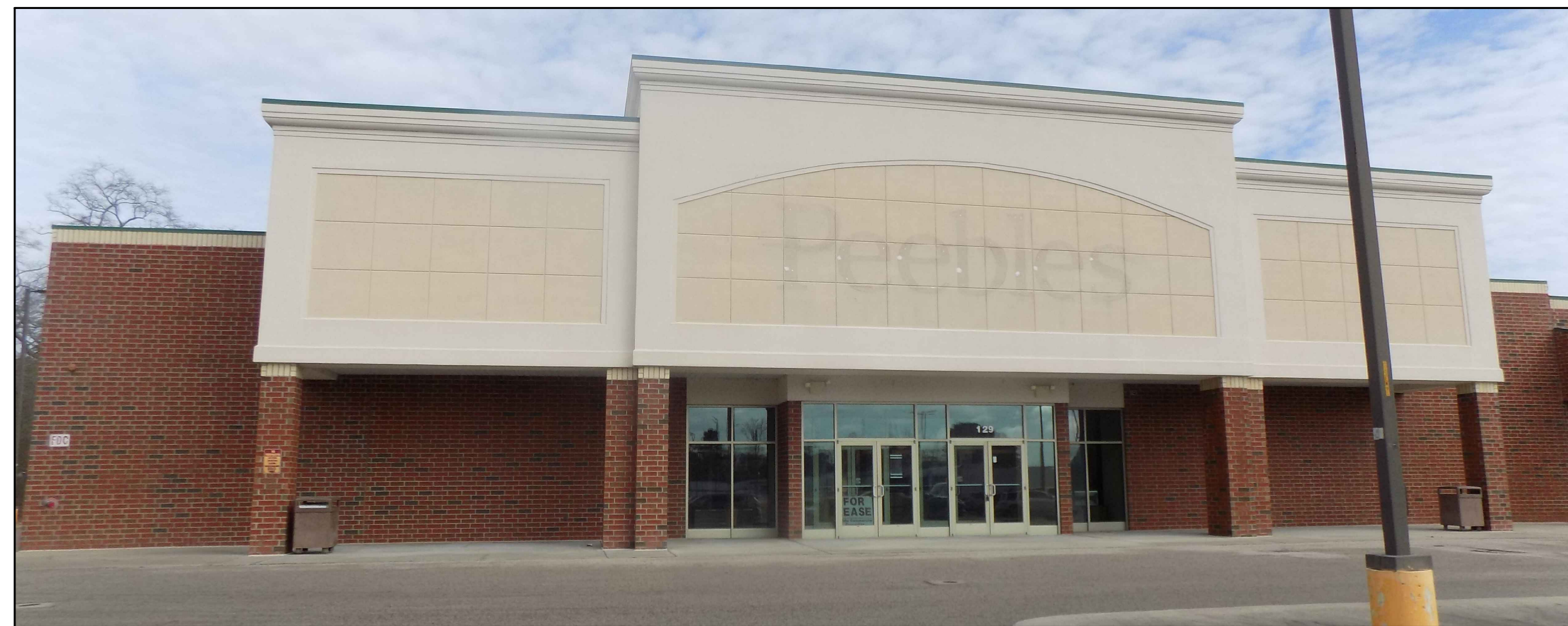
PHOTO OF EXISTING SOUTH ELEVATION
