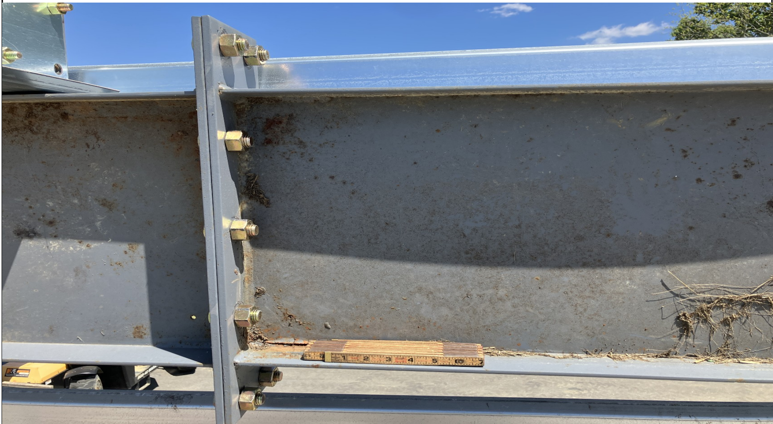
Photo 2 – Checking bolted connections on roof level framing
