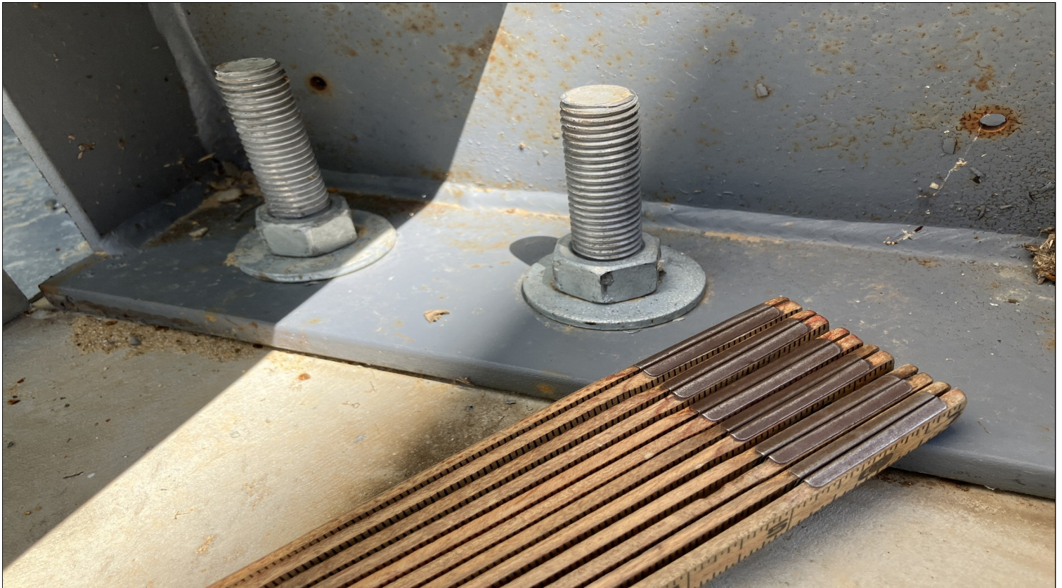
Photo 3 – Checking column anchors
