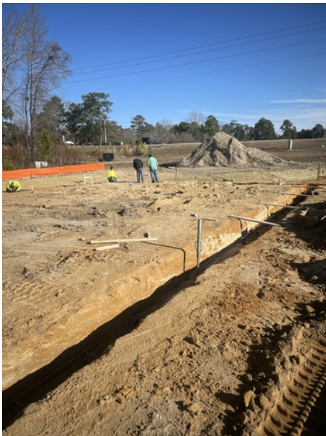
(P2) Building pad
