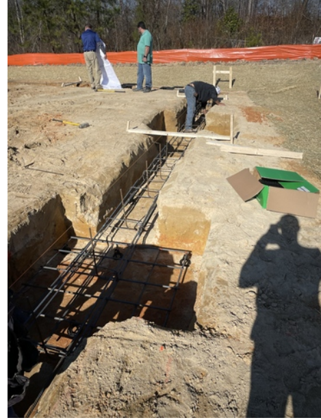
(P3) North east column footings
