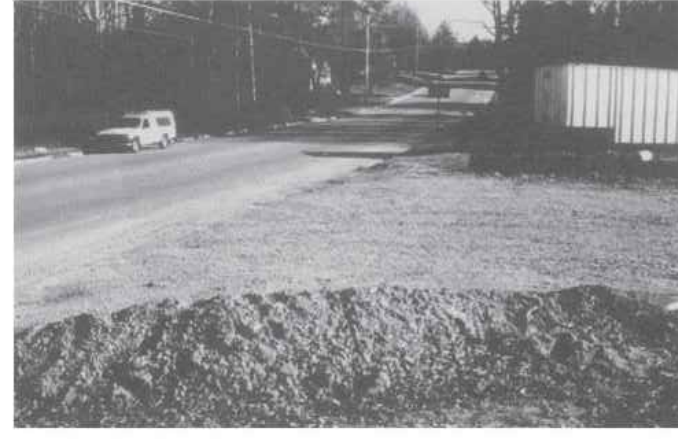
Figure 6.06a Gravel entrance/exit keeps mud off public roads.
