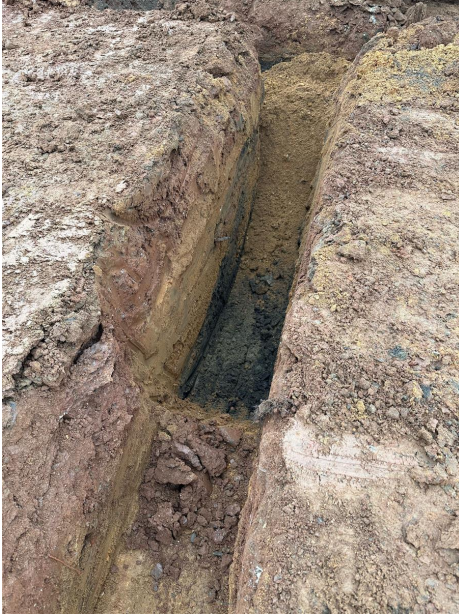
Topsoil and debris layer
