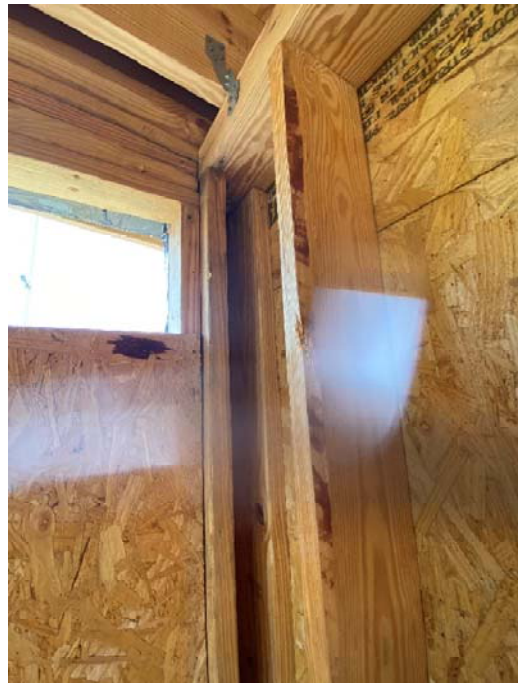
Figure 4: Another Corner stud that requires Blocking.
