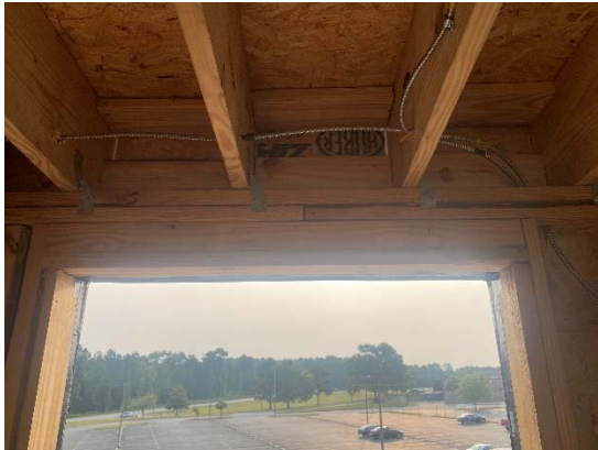
Figure 1: Door Header over East/West Wall.
