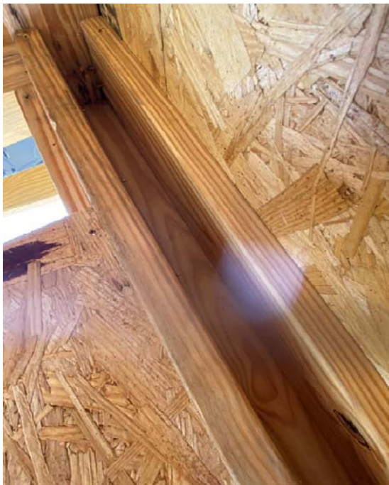
Figure 3: Corner stud that requires blocking.
