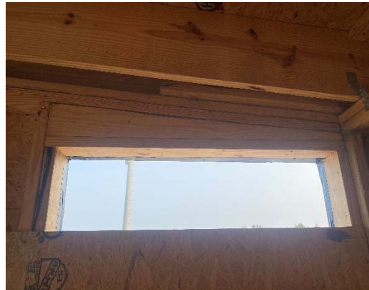
Figure 2: Header at endwall filled in solid.
