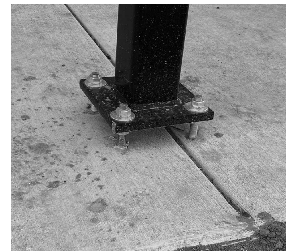
8 SUPPORT POST DETAIL NTS
