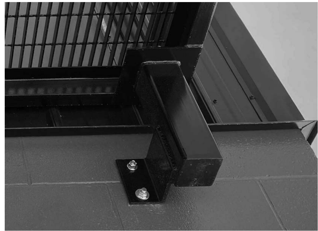
7 PLATFORM BRACKET CONNECTION NTS
