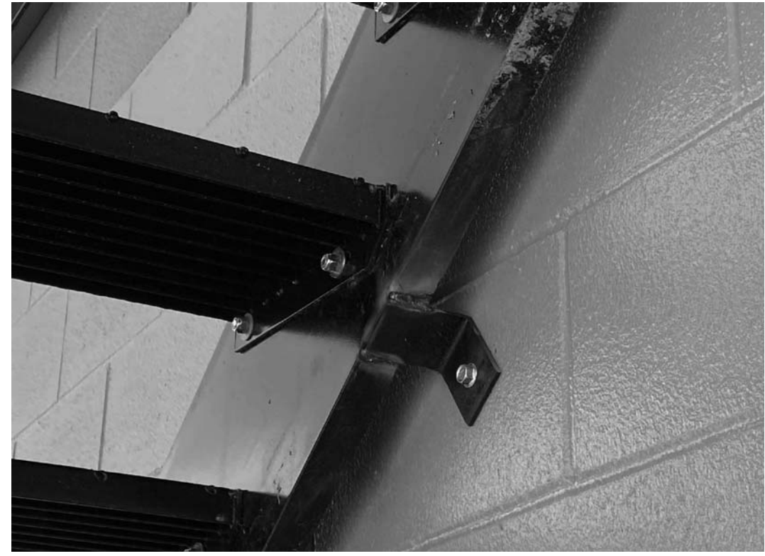
6 STAIR ANCHOR DETAIL NTS
