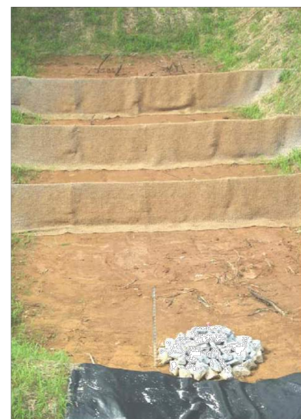
Figure 6.65c Example of porous baffles made of 700 g/m 2 coir erosion blanket as viewed from the outlet.
