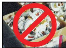
INCORRECT (Protective caps not in place)
