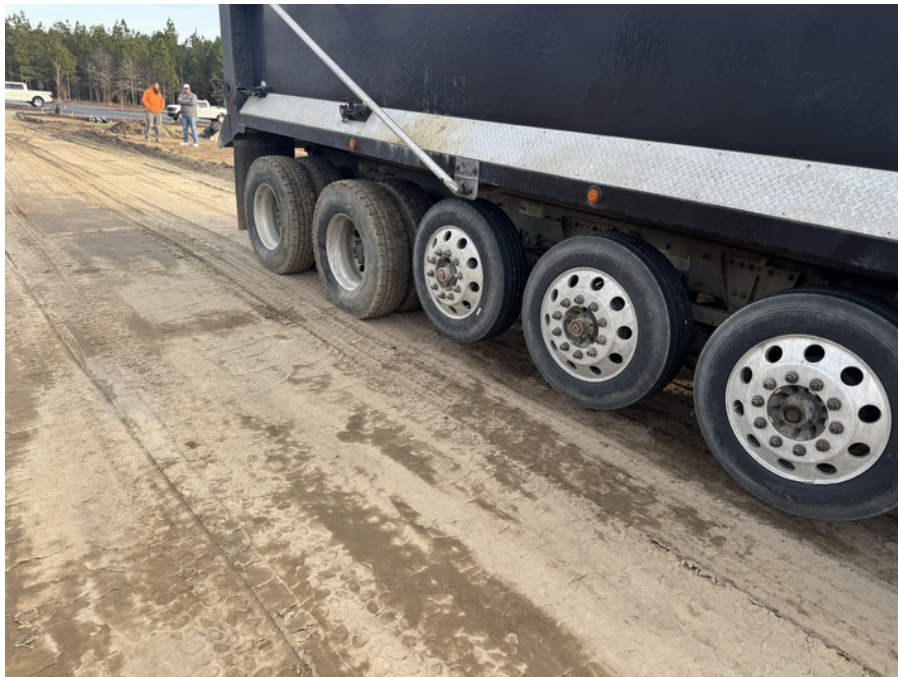
(P2) Proofroll in progress
