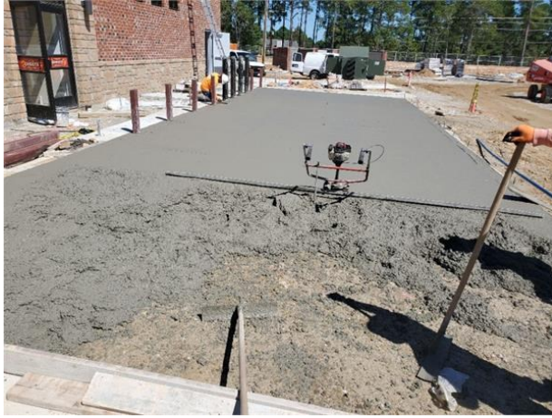
Concrete Placement
