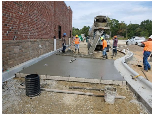
Concrete Placement @ Drive-Thru
