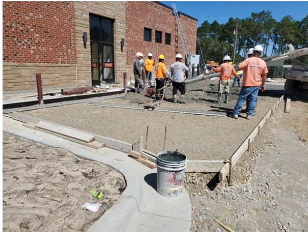
Concrete Placement
