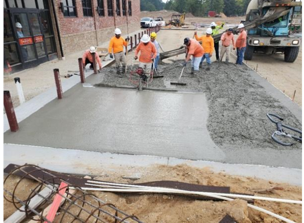
Concrete Placement & Consolidation Efforts
