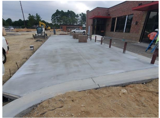
Concrete Pavement Area #6
