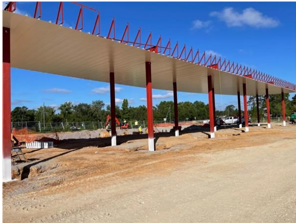
Gas Pump Canopy
