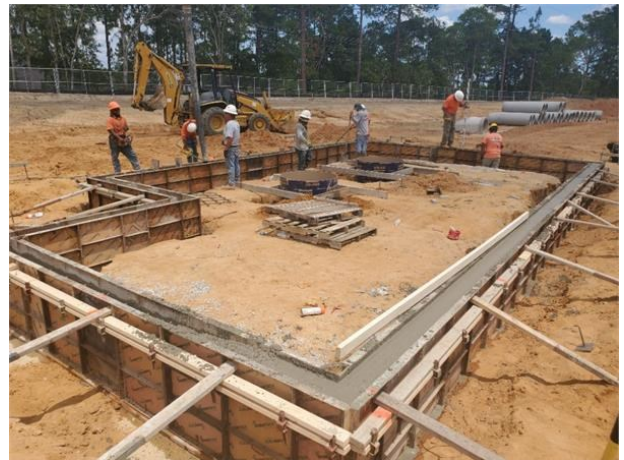
Concrete Placement
