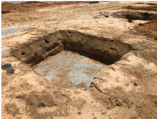
57 stone in footing B-3
