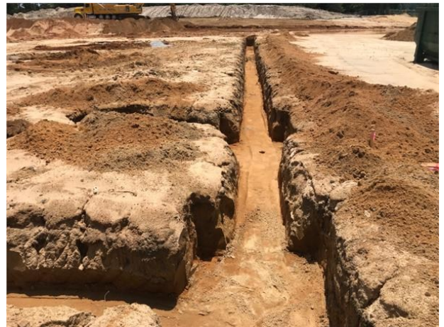
Excavated footing along line C
