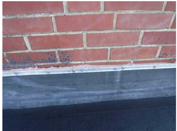
Photo #22 Non-asbestos Pink Roof Caulk (HA #20)
