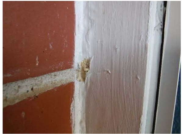
Photo #28 Non-asbestos Beige Window/Door Caulk (HA #30)
