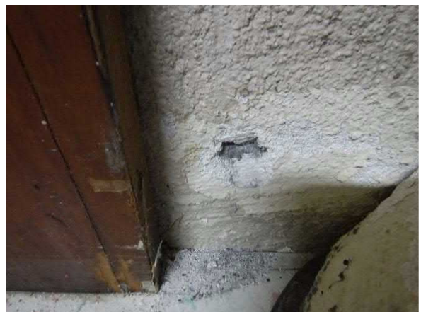
Photo #12 Non-asbestos CMU Skim Coat (HA #8)
