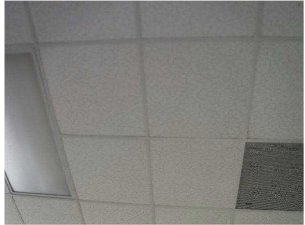
Photo #20 Non-asbestos 2'x2' Ceiling Tile (HA #18)
