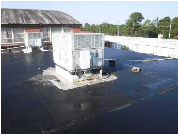
Photo #23 Non-asbestos Older White Roof Mastic (HA #21, foreground) and Newer White Roof mastic (HA #22, background)
