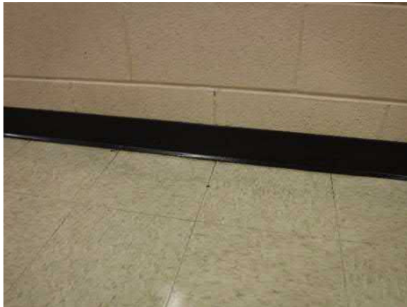
Photo #1 12"x12" Beige w/Brown Specks Floor Tile with Asbestos-Containing Mastic (HA #2) and Non-asbestos 4" Black Cove Base/Mastic (HA #6). Non-asbestos brown leveling compound (HA #7) located under tile.
