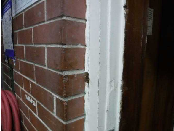
Photo #15 Non-asbestos Beige Interior Door Caulk (HA #12)
