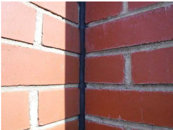
Photo #29 Non-asbestos Black Expansion Joint Caulk (HA #32)
