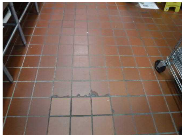
Photo #10 Non-asbestos Red Ceramic Floor Grout and Mastic (HA #4)
