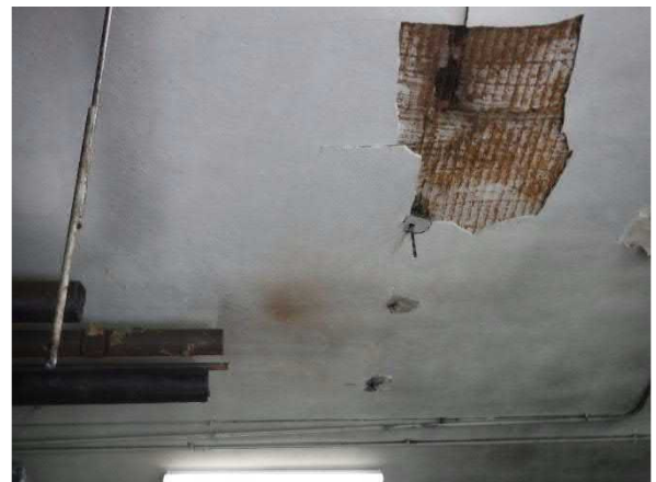
Photo #18 Non-asbestos Plaster Brown Coat (HA #15)
