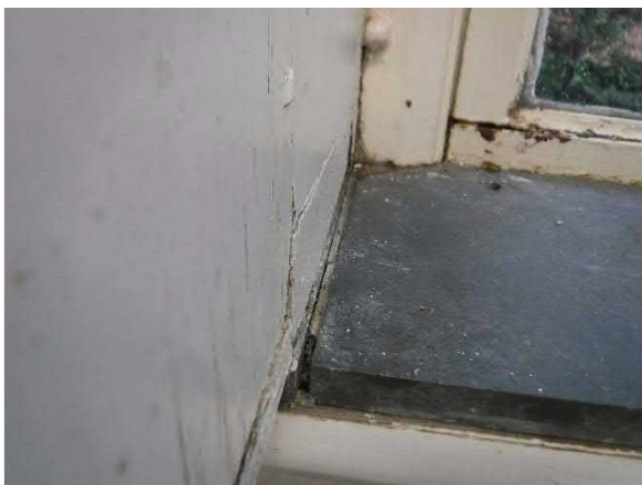
Photo #11 Non-asbestos Grey Window Sill Grout (HA #5)
