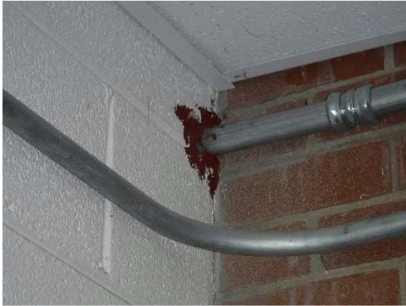
Photo #25 Non-asbestos Red Fire Caulk (HA #26)
