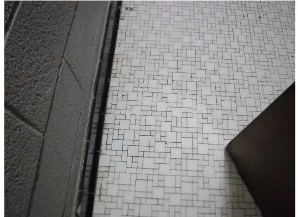
Photo #14 Non-asbestos White Ceramic Grout and Mortar (HA #11)
