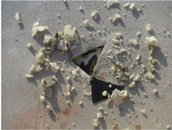
Photo #19 Non-asbestos Foam Insulation Paper Backing (below membrane) (HA #16)
