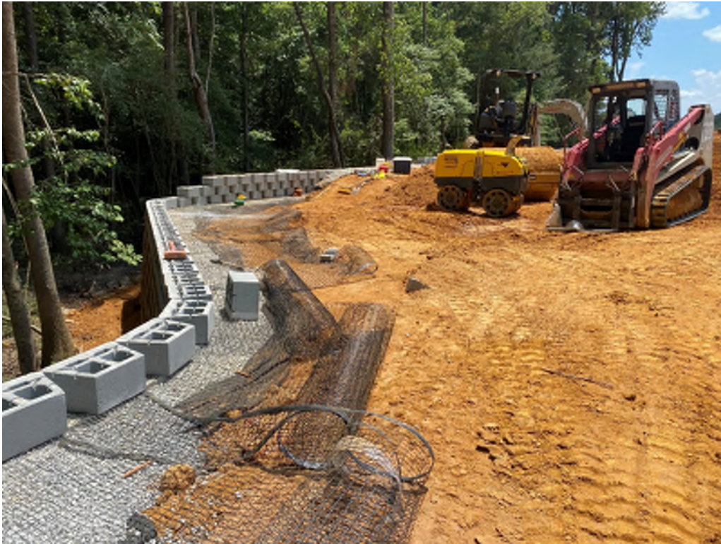
Figure 1: Installing geogrid from approximately 3+50 – 4+80.
