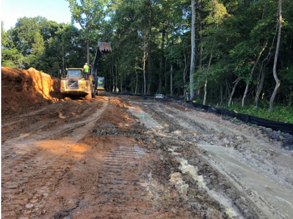
Figure 1: A trackhoe removes wet soil from the wall area.
