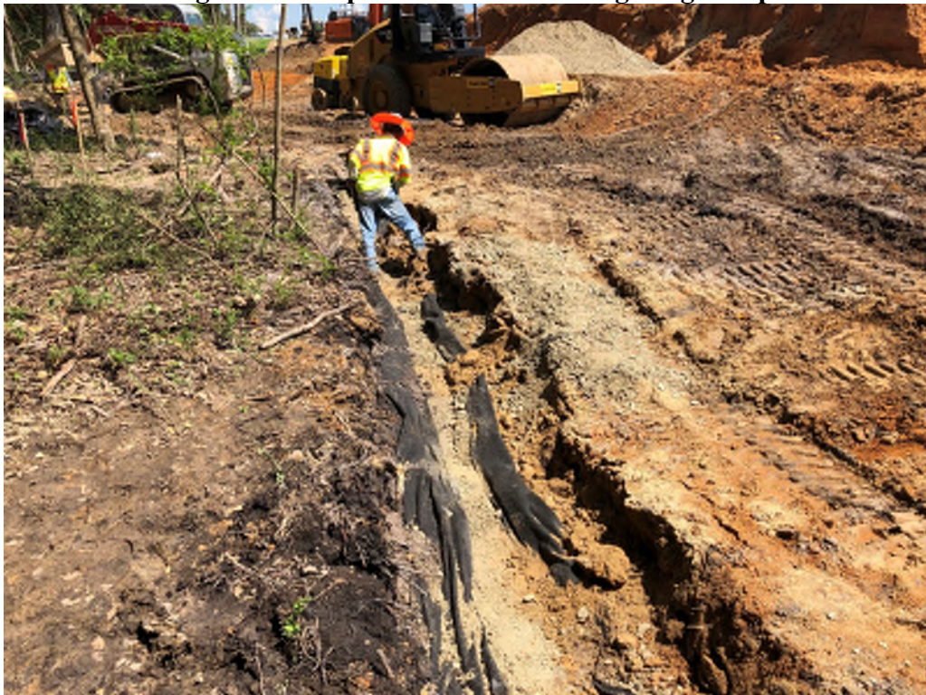
Figure 7: A jumping jack is used to compact the ABC stone base.
