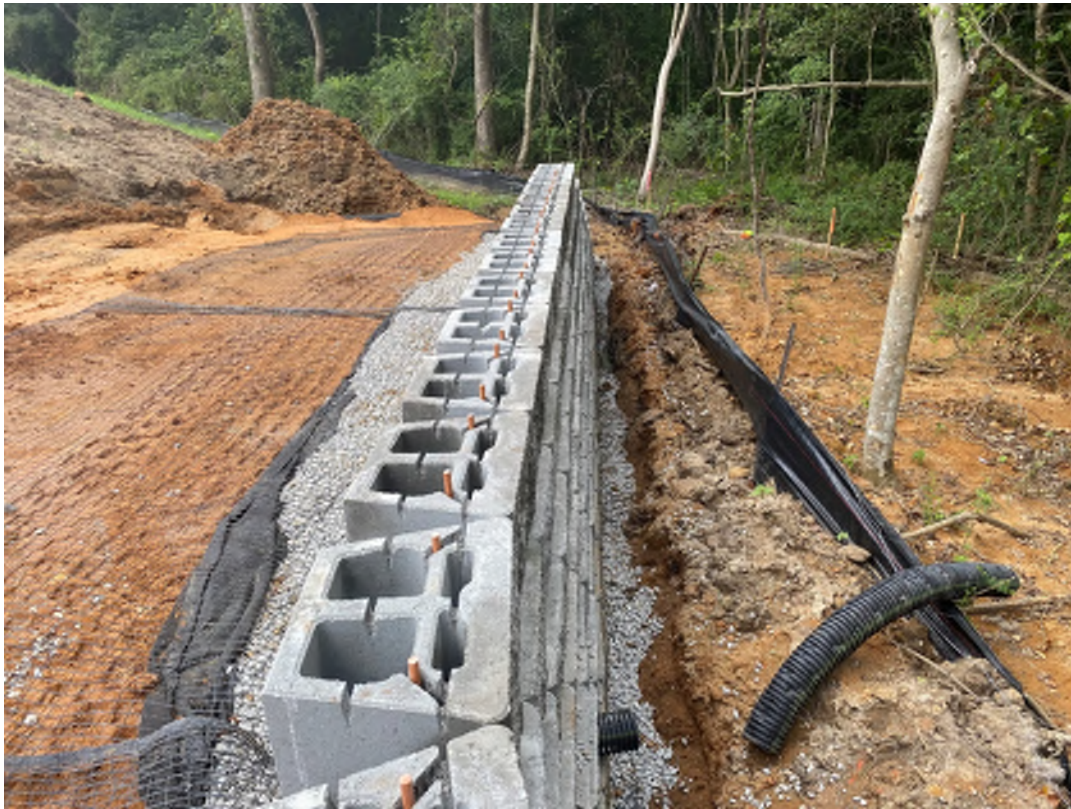
Figure 4: Wall construction at approximately 4+50.
