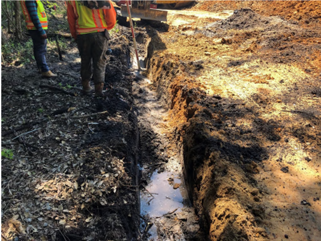
Figure 4: Excavating the footer for the retaining wall.
