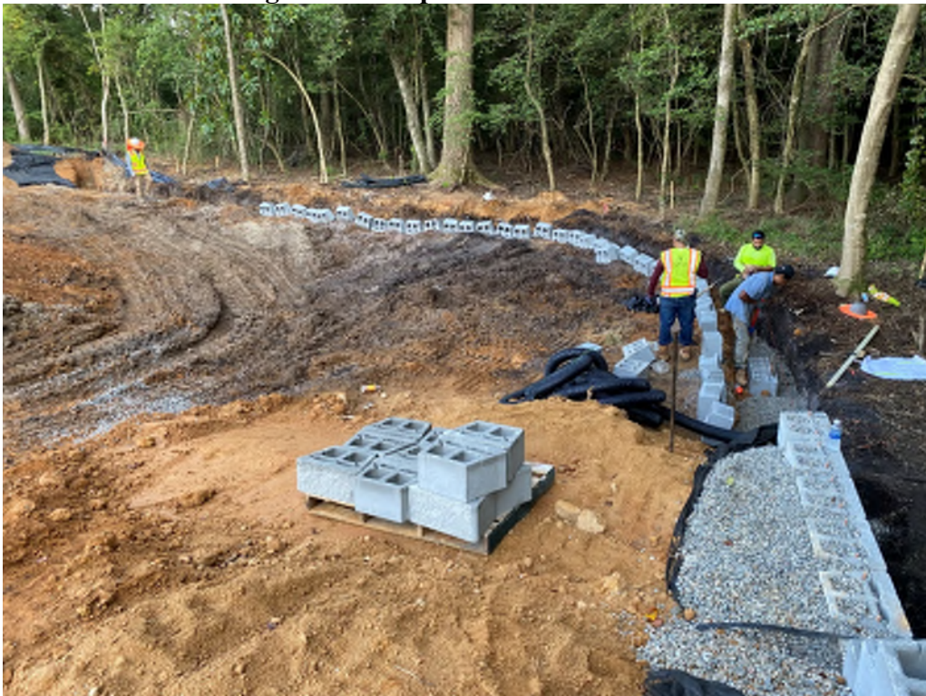
Figure 3: Retaining wall from 3+50 to 4+80.
