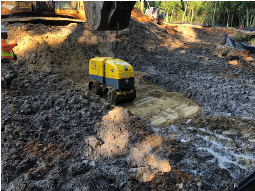
Figure 3: An RC trench roller is used to backfill the undercut area.
