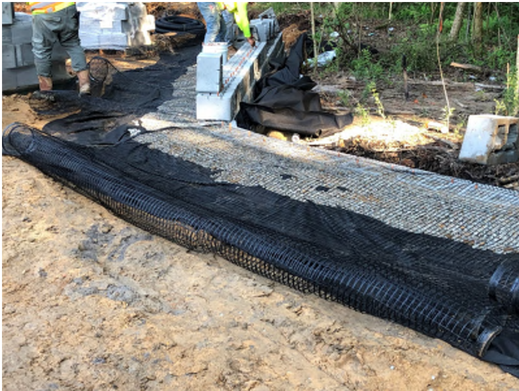
Figure 1: Geogrid installation at approximately ST 3+60
