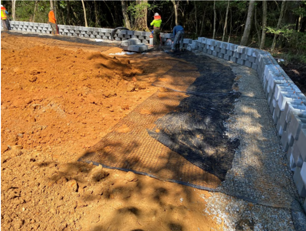
Figure 1: Installing geogrid from approximately 3+70 – 4+80.
