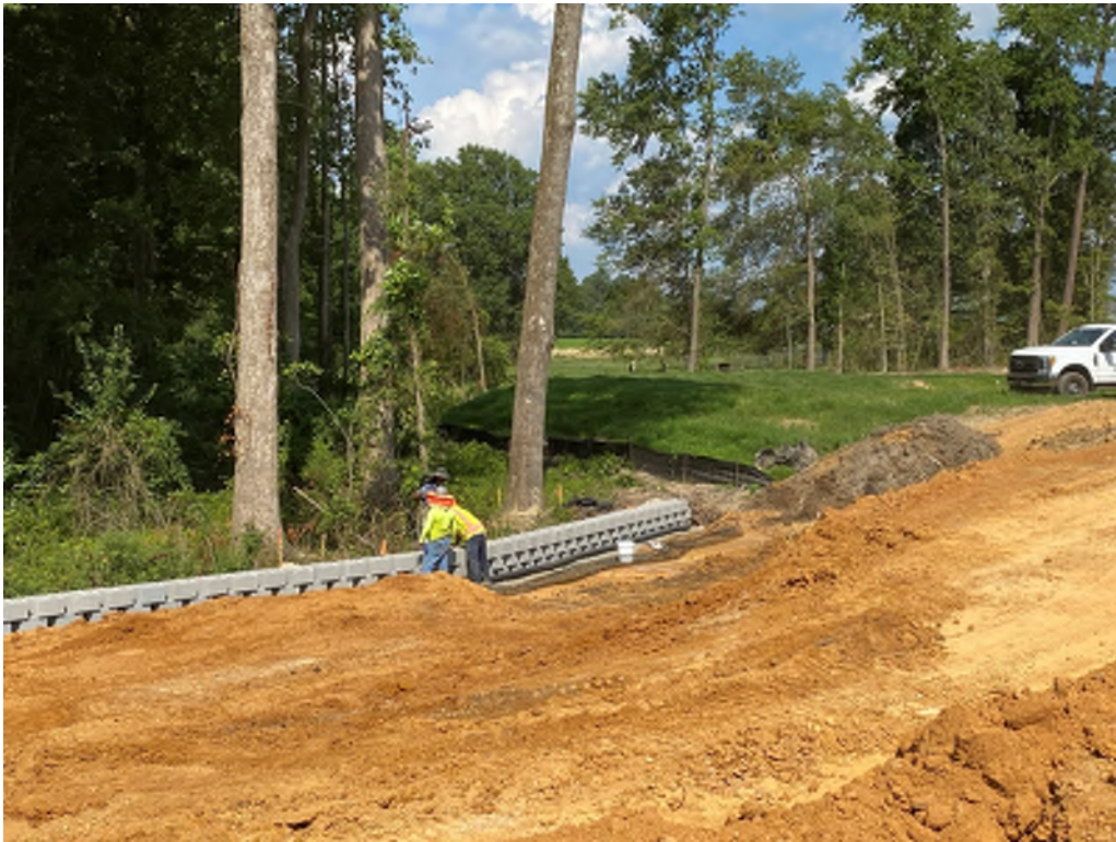
Figure 2: Wall construction at 0+00.
