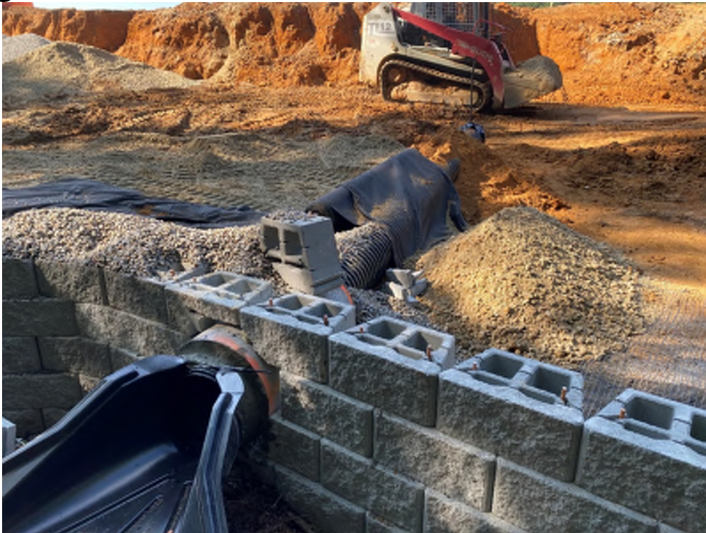
Figure 1: 12" storm drain installed with concrete collar at approximately 3+76.
