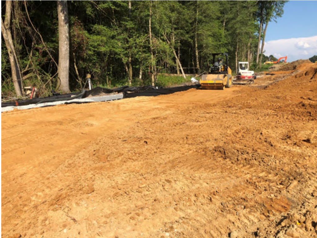
Figure 4: Backfill is compacted utilizing a smooth drum roller.
