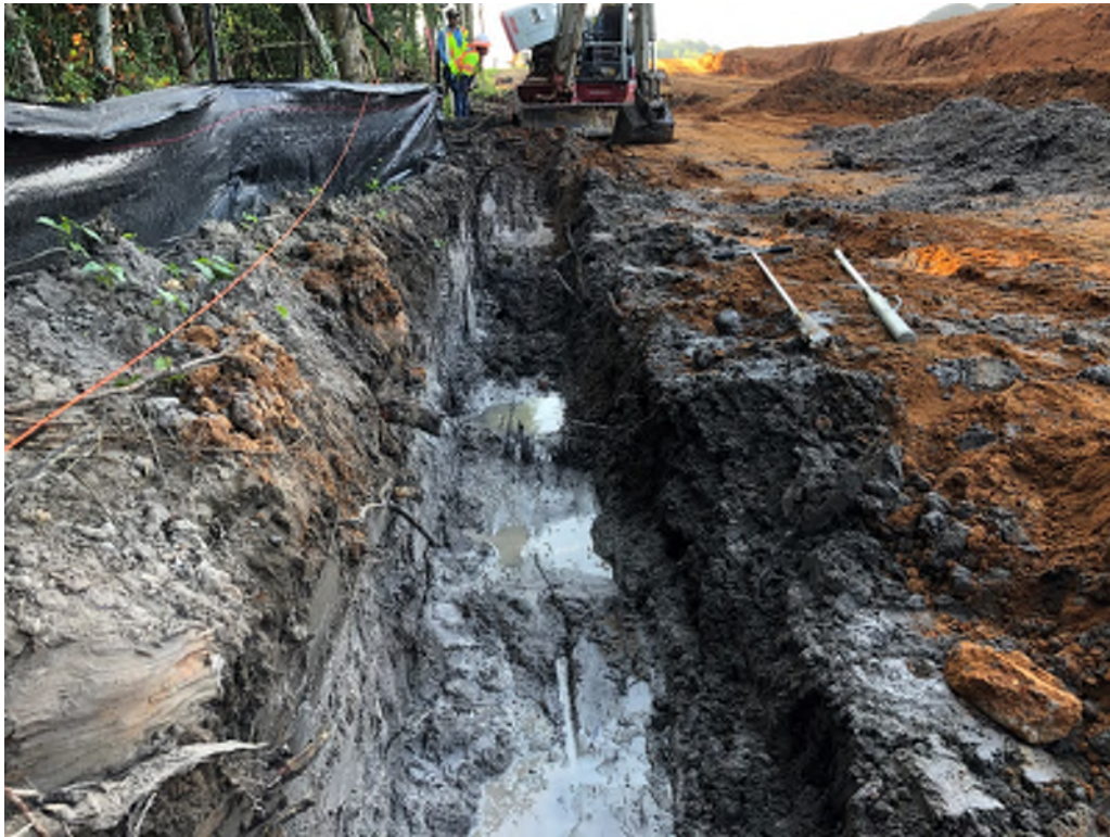
Figure 2: Excavated footings at ST 1+50
