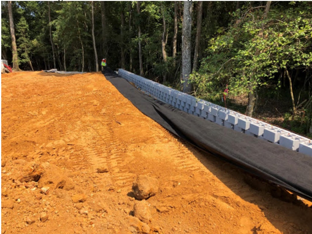
Figure 3: Separation geotextile
