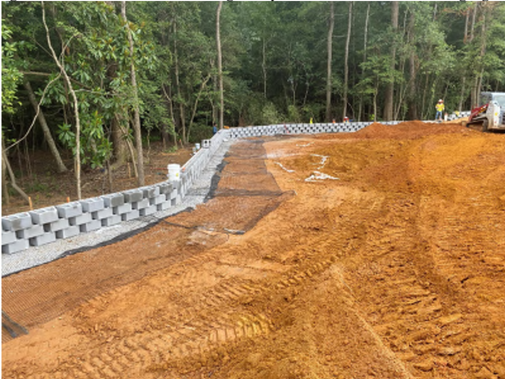
Figure 3: Retaining wall from 3+50 to 4+80.
