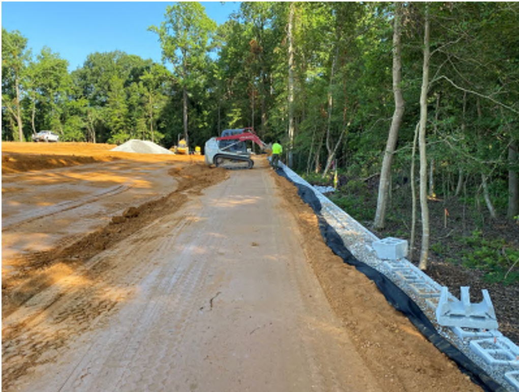
Figure 2: Compacted reinforced soil.
