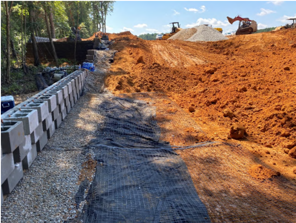
Figure 2: Geotextile fabric showing 2' key into reinforced soil under geogrid.
