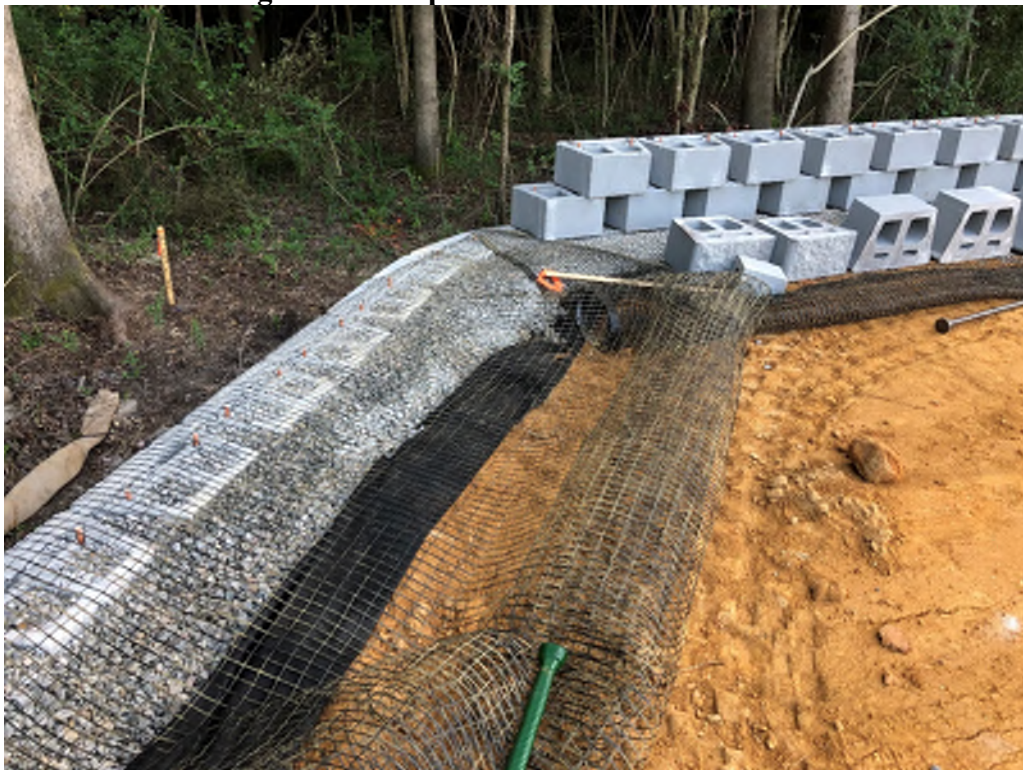
Figure 5: Geotextile is placed over the fiberglass pins
