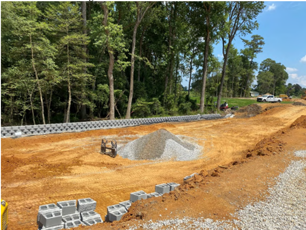
Figure 3: Retaining wall from 1+50 to 0+00.
