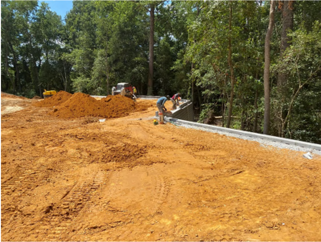
Figure 2: Vertical walls installing the Capstones upon meeting final elevation from 3+35 to 4+80.
