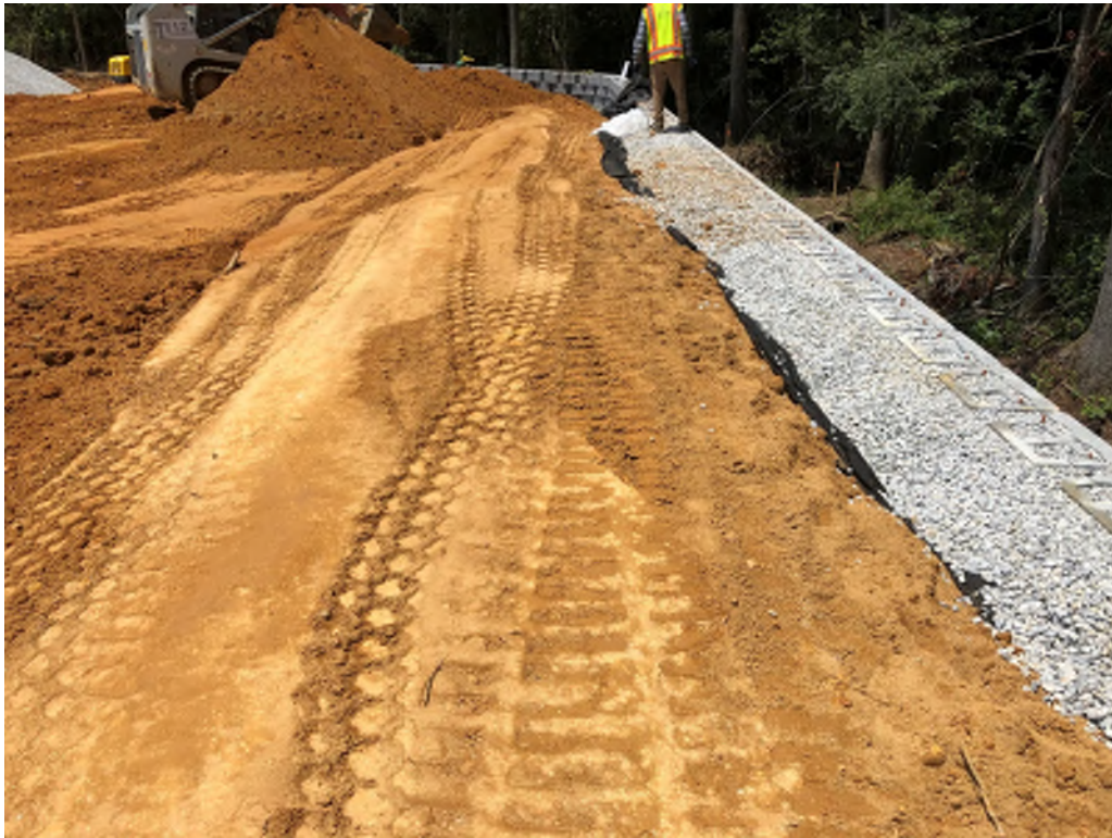
Figure 4: Compacted reinforced zone soils
