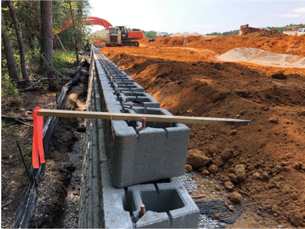
Figure 2: Wall construction facing towards ST 2+00
