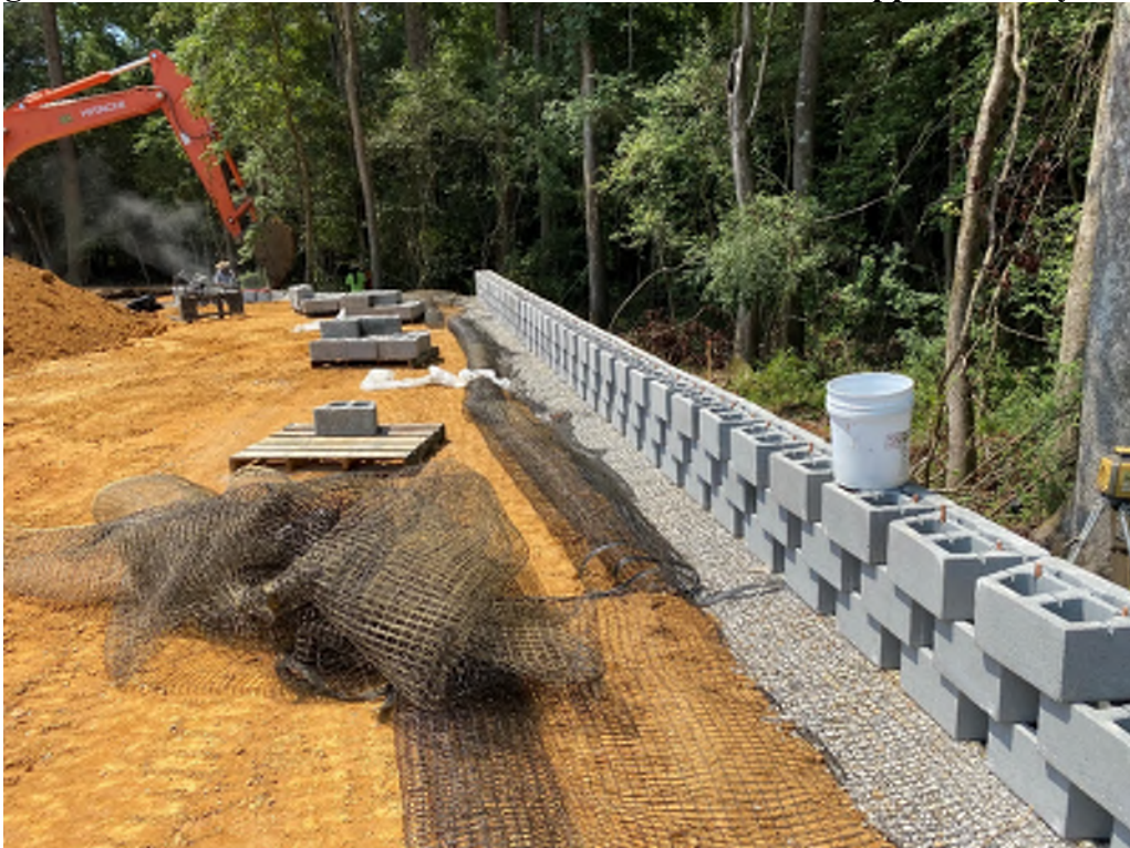
Figure 3: geogrid installation at approximately 2+25.
