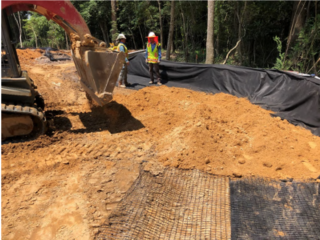
Figure 6: Placing a lift of soil backfill.
