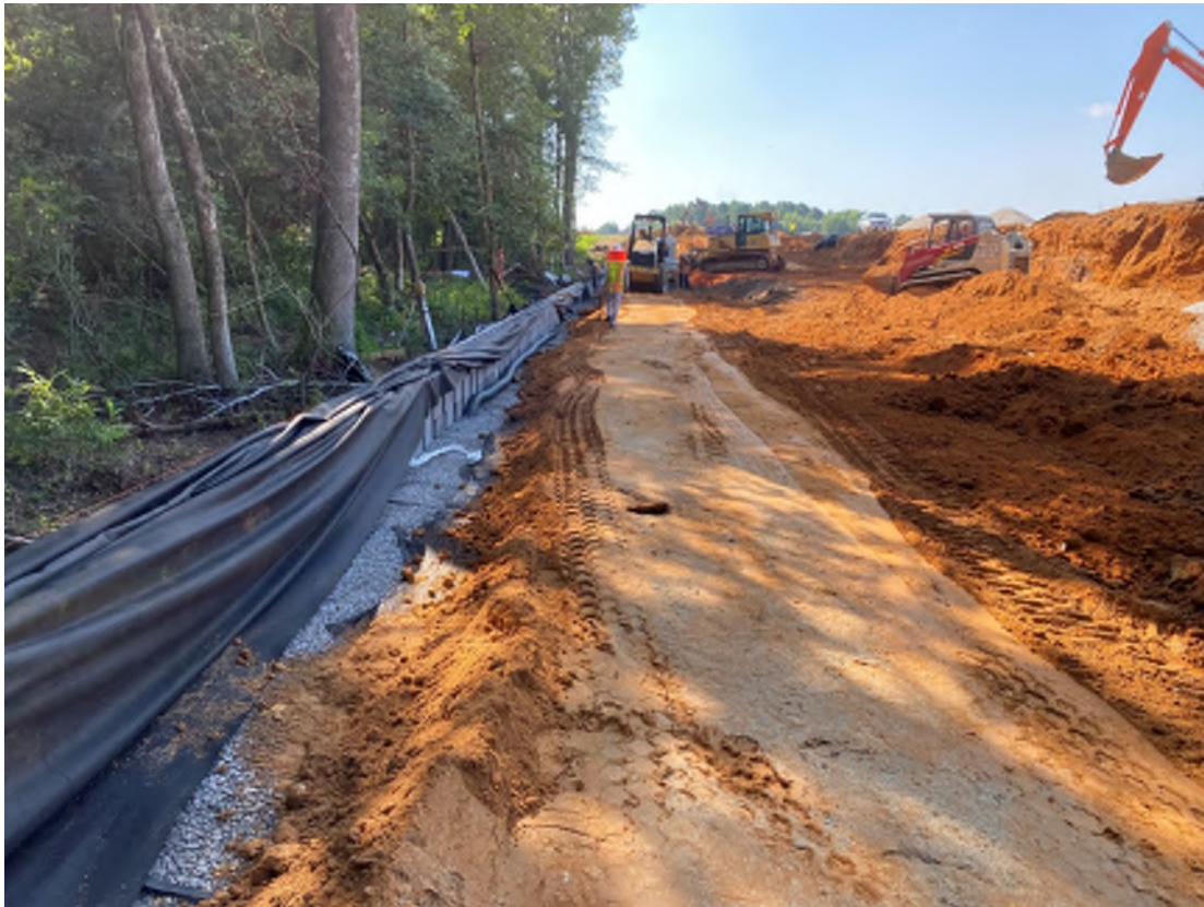
Figure 4. Vertical Walls compacting backfill over geogrid.
