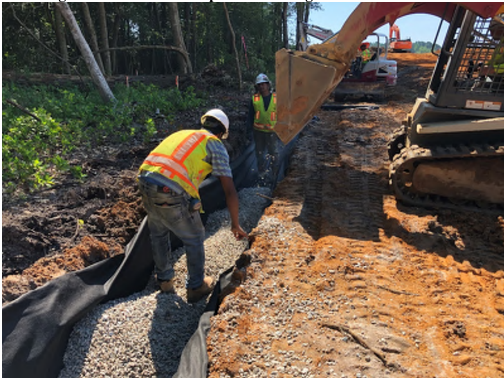
Figure 5: Installing geotextile wrapped #57 stone for the wall footing.
