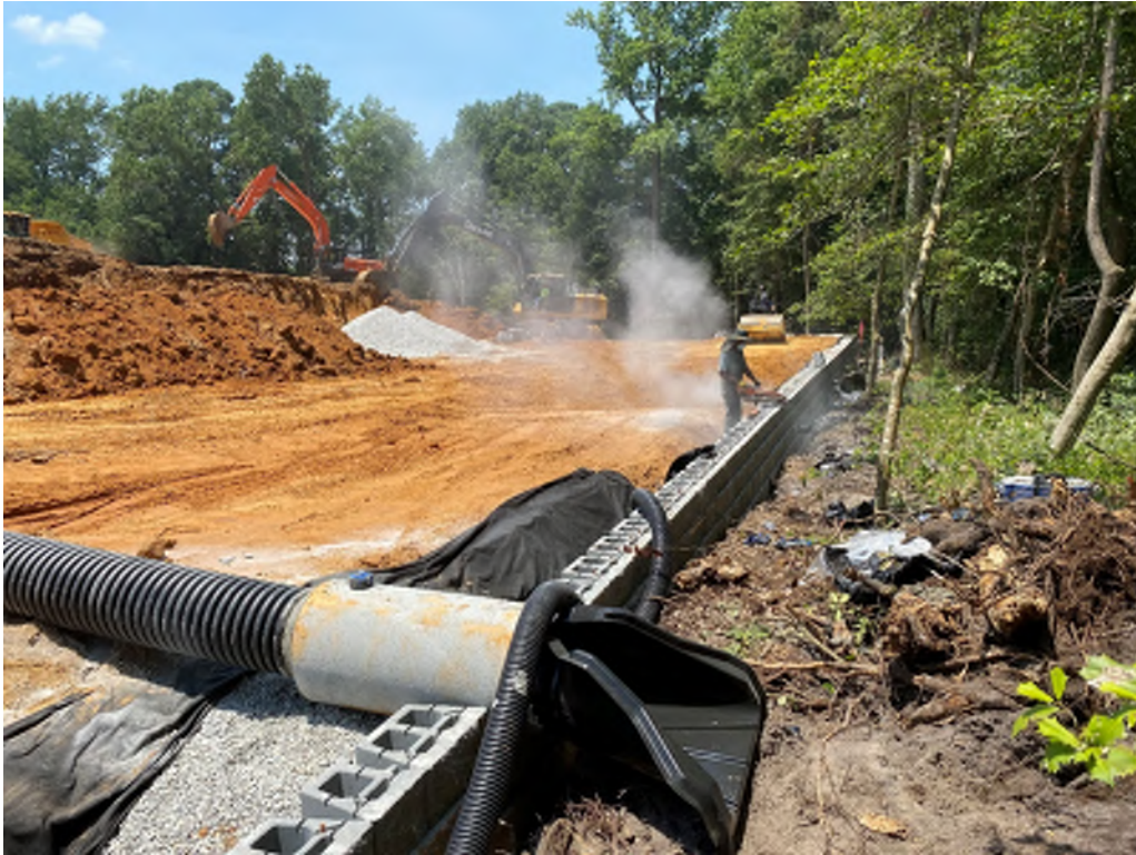
Figure 2: 12" storm drain installed with concrete collar at approximately 1+75.
