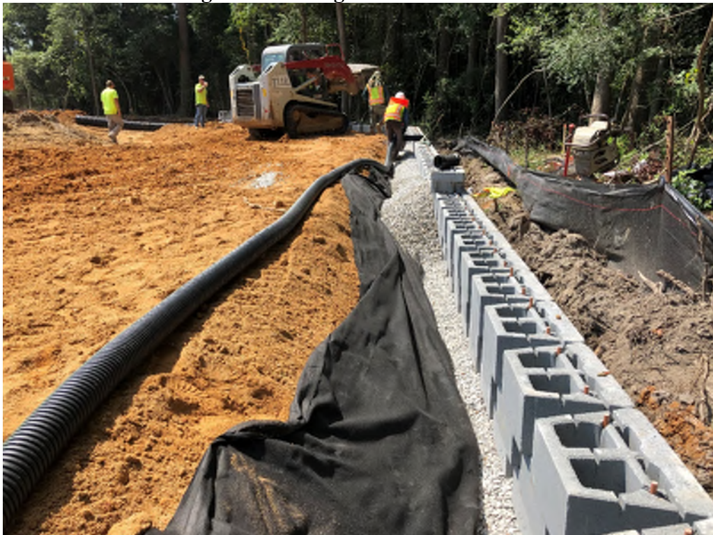
Figure 7: Installing drainage layer and the 4" perforated through drains.
