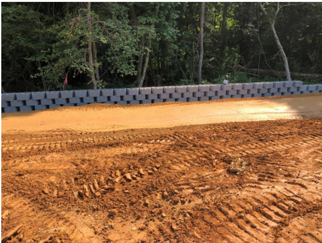
Figure 1: Compacted fill within the reinforced zone.
