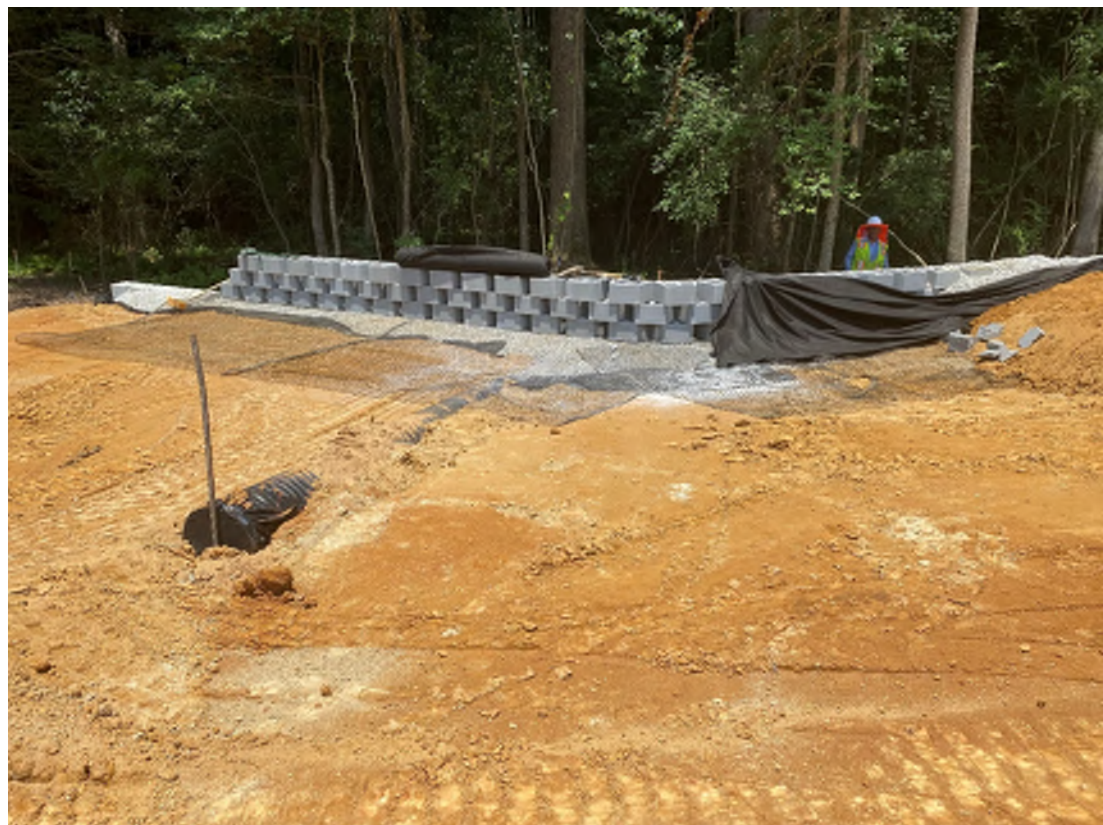
Figure 5: 12" CPP at approximately ST 3+76.
