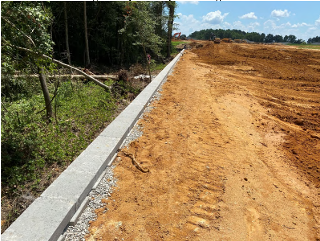
Figure 3: Capstones in place from 3+20 facing 0+00.
