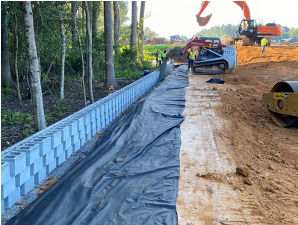
Figure 1: Installing the last lift of drainage layer from ST 0+00 to 3+00.
