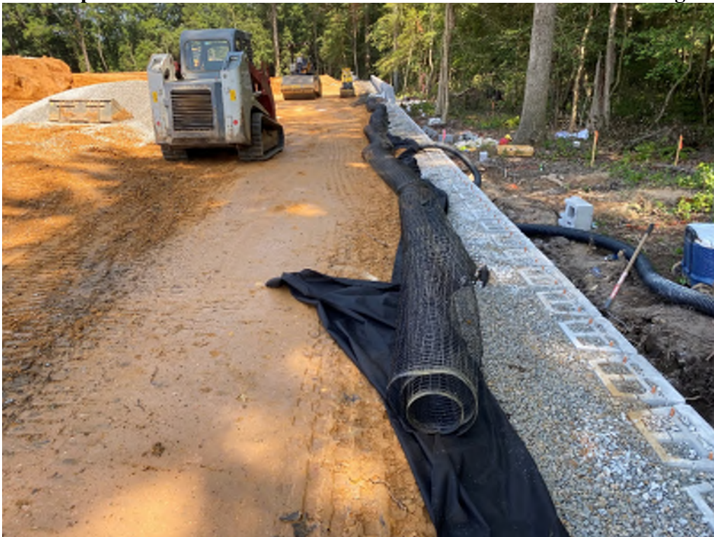
Figure 5: Geogrid is being staged ready for installation.
