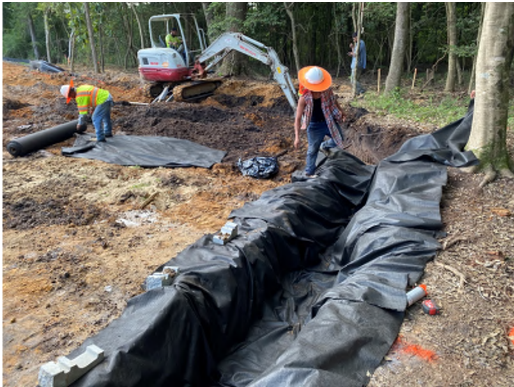
Figure 1: Footer excavation from ST 3+75 – 4+80.
