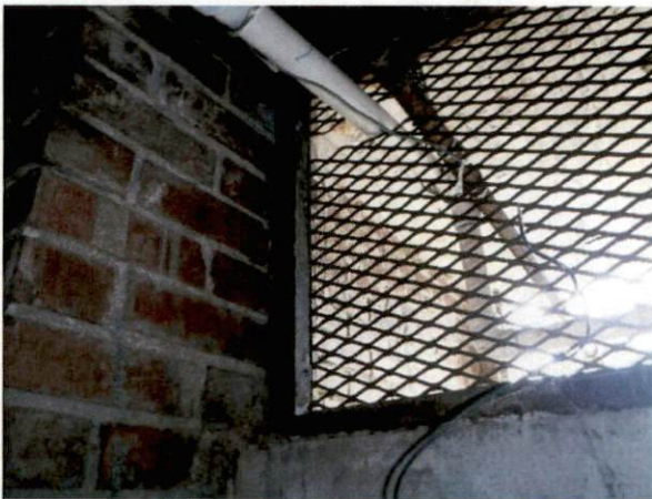
Photo #15 View of boiler window with HA 7, asbestos-containing interior window glazing.
