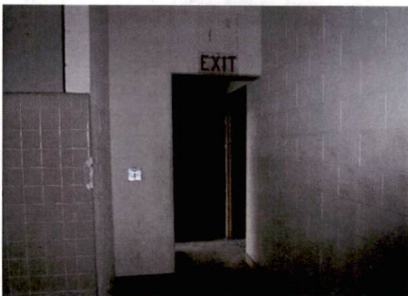
Photo #23 View of HA 19, non-asbestos containing CMU block filler.
