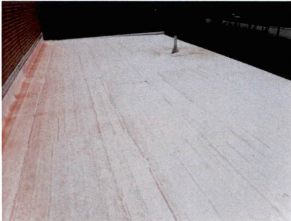
Photo #7 View of west roof.
