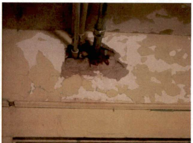
Photo #18 View of HA 10, non-asbestos containing red firestop.
