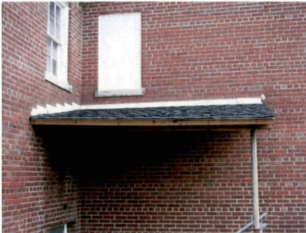
Photo #39 View of HA 34, non-asbestos containing black shingles and felt paper.
