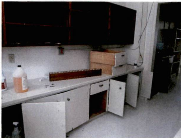
Photo #3 View of office area.
