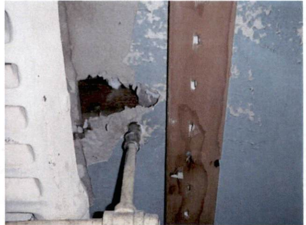
Photo #20 View of HA 12, non-asbestos containing plaster over non-asbestos containing drywall lathe.
