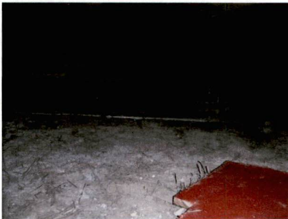
Photo #5 View of crawlspace.
