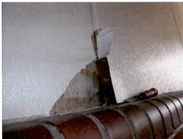
Photo #13 View of HA 9, non-asbestos containing beige FRP adhesive.
