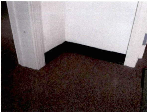
Photo #33 View of HA 27, non-asbestos containing 4" black cove base and mastic.
