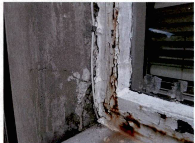
Photo #22 View of HA 16, non-asbestos containing white exterior caulk.
