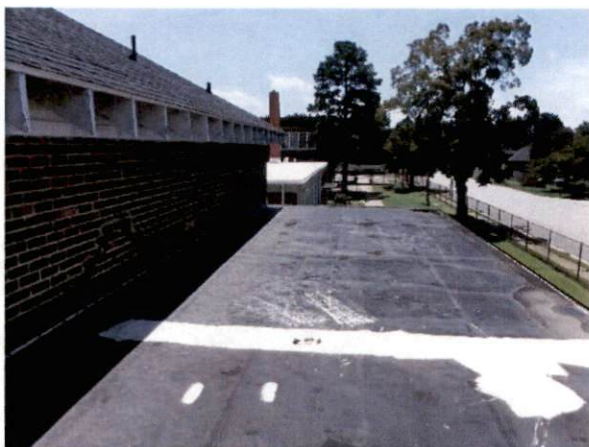
Photo #11 View of west roof.
