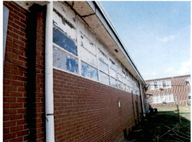
Photo #14 View of exterior with HA 7, non-asbestos containing textured exterior soffit.
