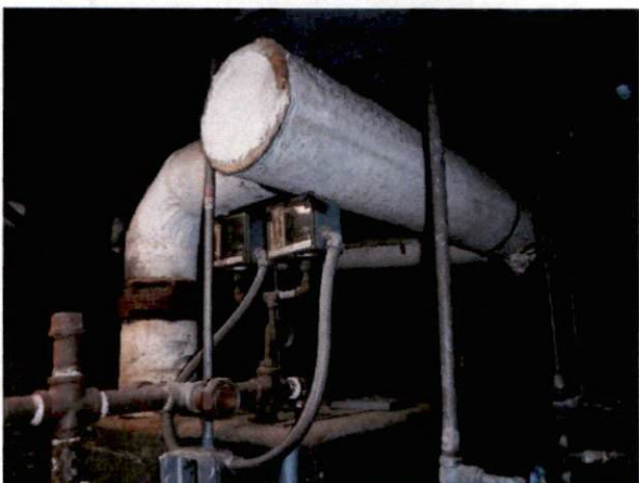
Photo #11 View of HA 4, non-asbestos containing white mud TSI joint.
