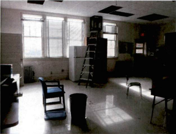
Photo #3 View of classroom.
