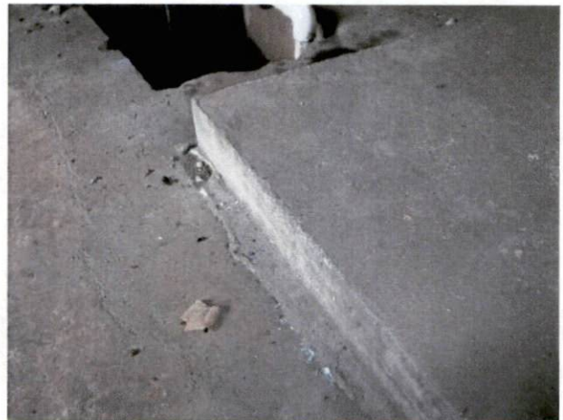
Photo #14 View of HA 6, non-asbestos containing lightweight concrete.
