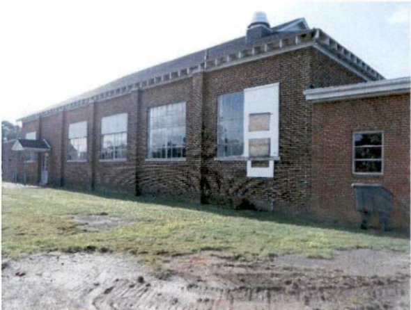
Photo #1 View of building exterior.
