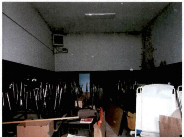
Photo #6 View of northeast storage room.
