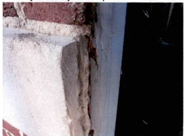
Photo #30 View of HA 26, non-asbestos containing red exterior door caulk.
