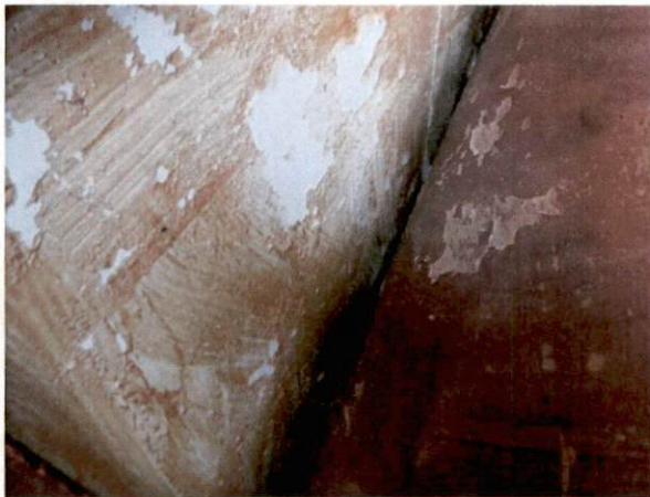
Photo #27 View of HA 21, non-asbestos containing tan glue behind plastic panel.
