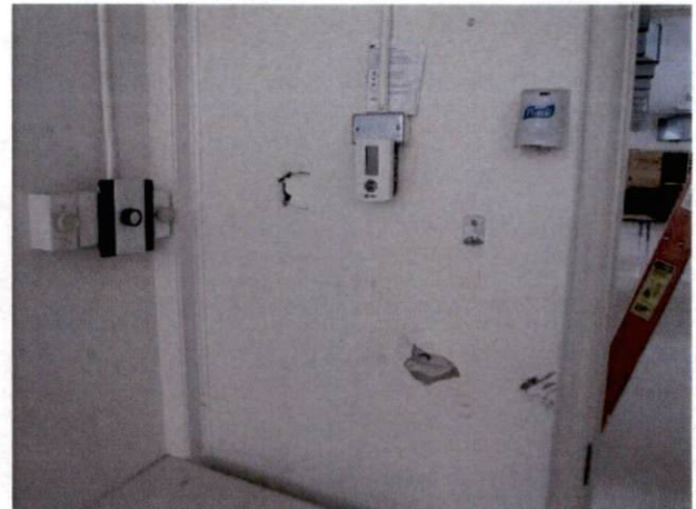
Photo #20 View of HA 14, non-asbestos containing drywall.
