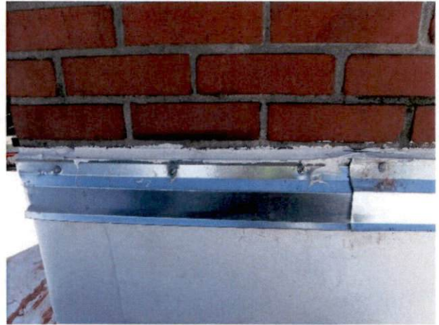
Photo #8 View of HA 1, non-asbestos containing white roof caulk.
