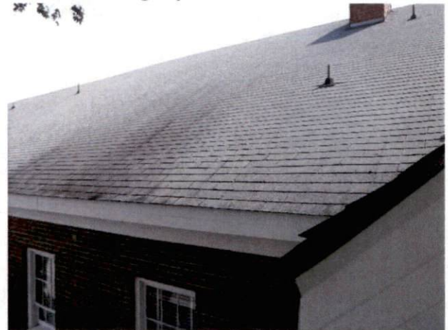
Photo #22 View of HA 14, non-asbestos containing gray shingles and felt paper.
