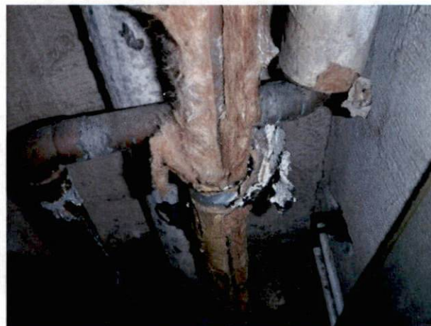
Photo #22 View of HA 16, non-asbestos containing black mastic on foil-backed paper over fiberglass pipe insulation.
