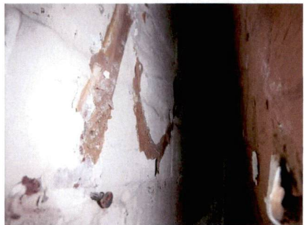
Photo #36 View of HA 31, non-asbestos containing brown FRP mastic.
