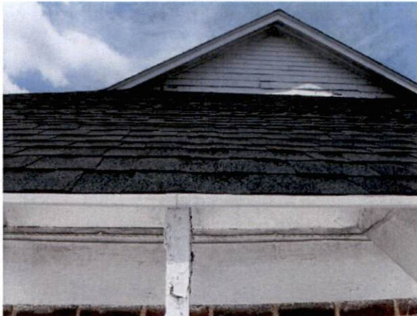
Photo #9 View of HA 3, non-asbestos-containing black shingles and felt paper.
