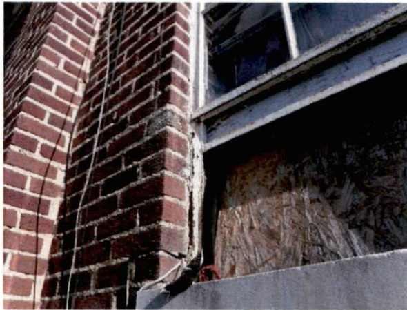
Photo #33 View of HA 27, non-asbestos containing exterior window caulk at brick.
