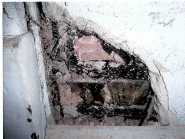
Photo #14 View of HA 10, non-asbestos containing black waterproofing.
