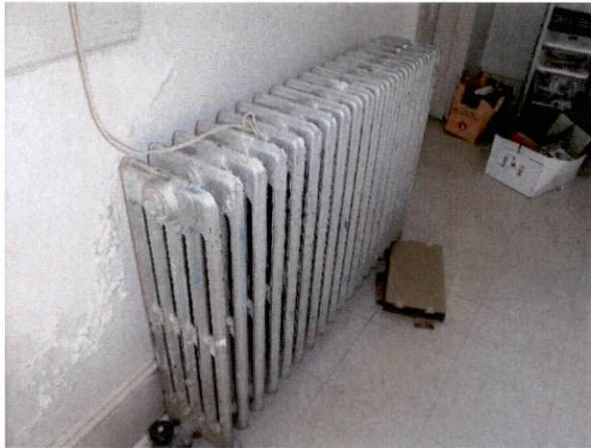
Photo #31 View of radiator with HA 25, non-asbestos containing silver paint.
