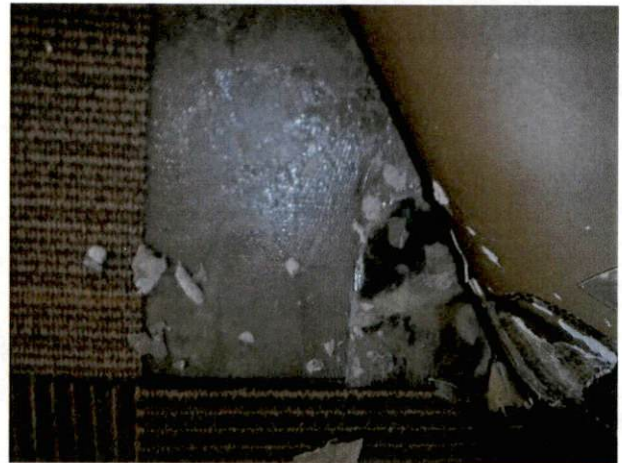
Photo #20 View of HA 16, non-asbestos containing gray leveling compound.
