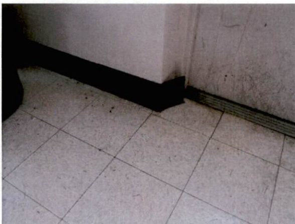
Photo #17 View of HA 10, non-asbestos containing 6" black cove base and mastic.
