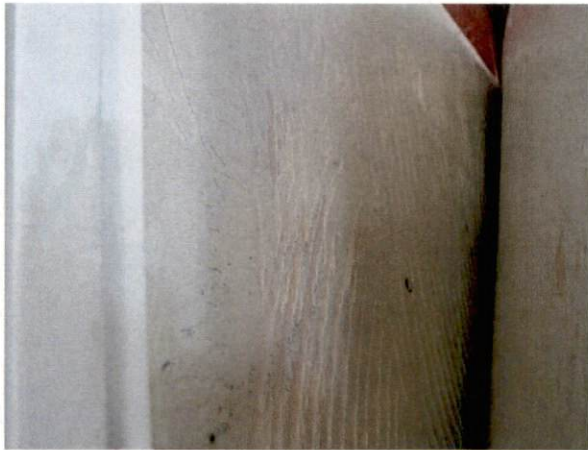
Photo #25 View of HA 19, non-asbestos containing beige FRP mastic.
