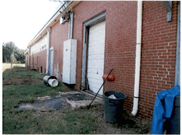
Photo #2 View of east exterior.
