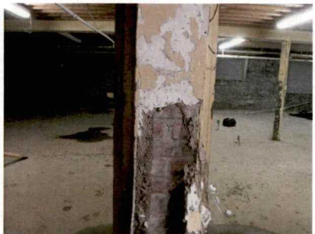
Photo #16 View of HA 8, non-asbestos containing plaster.
