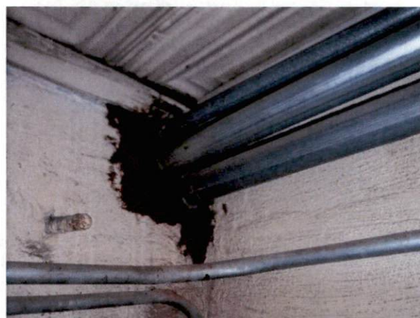
Photo #24 View of HA 18, non-asbestos containing dark red fire caulk.
