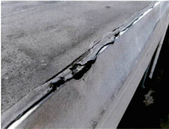
Photo #13 View of HA 6, non-asbestos containing black roof caulk on southwest roof.
