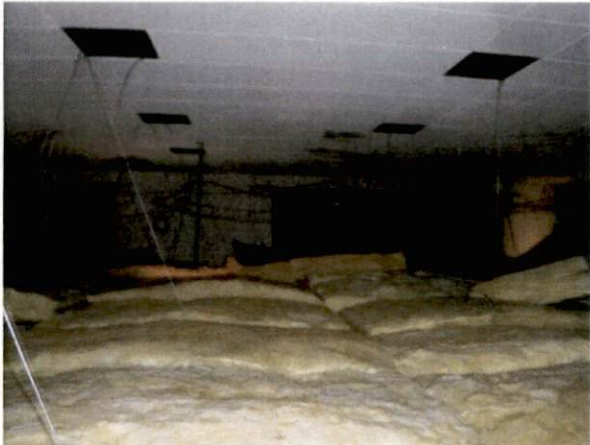
Photo #3 View of ceiling plenum.
