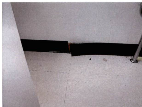
Photo #17 View of HA 13, non-asbestos containing 4" black cove base and mastic.
