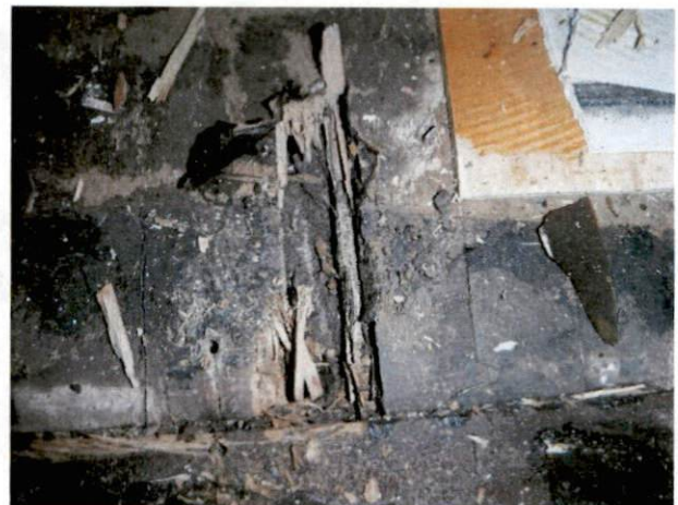
Photo #26 View of HA 19, non-asbestos containing black felt paper under hardwood flooring.
