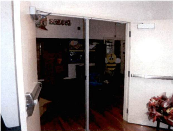
Photo #3 View of foyer.
