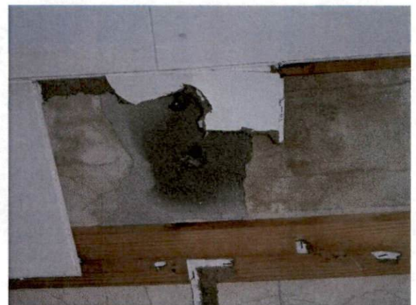
Photo #12 View of HA 8, non-asbestos containing textured plaster.
