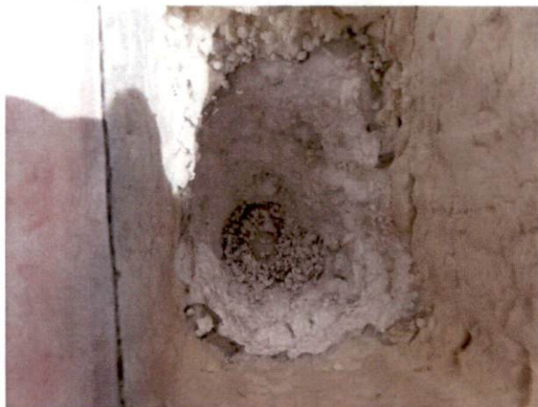
Photo #11 View of HA 4, non-asbestos containing lightweight concrete.
