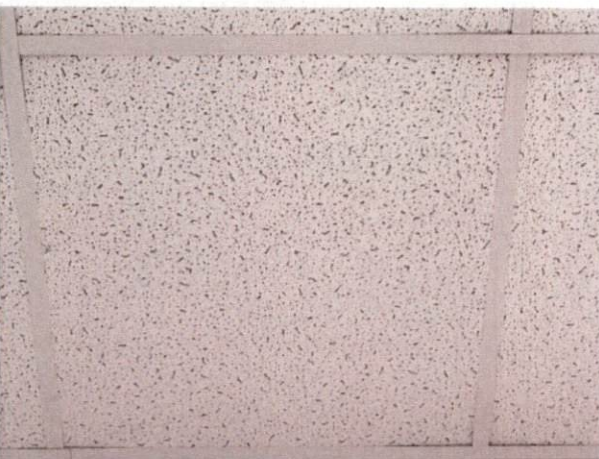
Photo #23 View of HA 19, non-asbestos containing 2' x 2' ceiling tile with dots and fissures.
