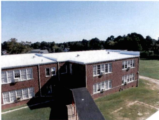
Photo #6 View of roof.
