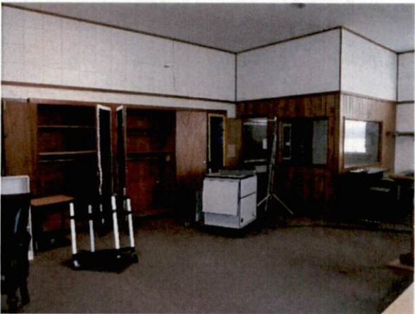
Photo #5 View of band room.
