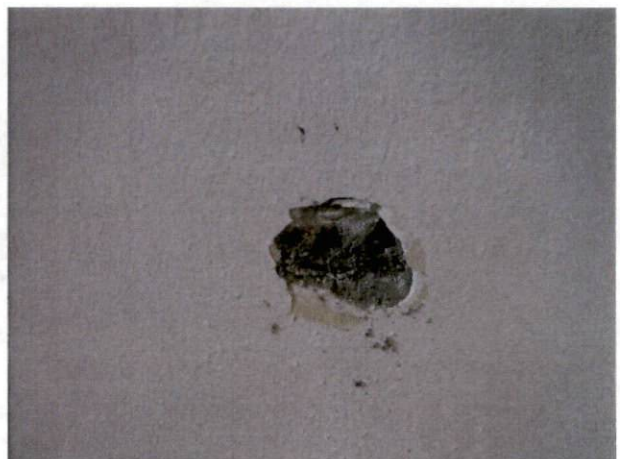
Photo #18 View of HA 11, non-asbestos containing plaster.
