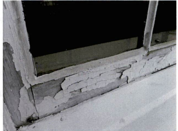
Photo #38 View of HA 33, non-asbestos containing exterior window glazing.
