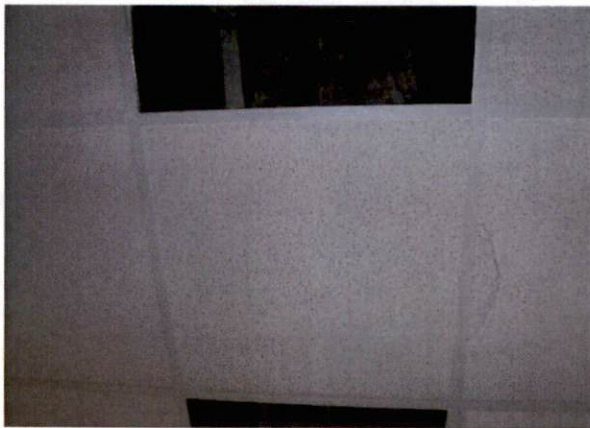
Photo #21 View of HA 17, non-asbestos containing 2' x 2' white ceiling tile with dots.
