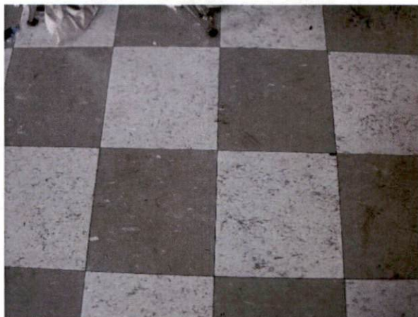
Photo #21 View of HA 15, asbestos-containing checkered 12" x 12" beige with brown specks/green floor tile and mastic.
