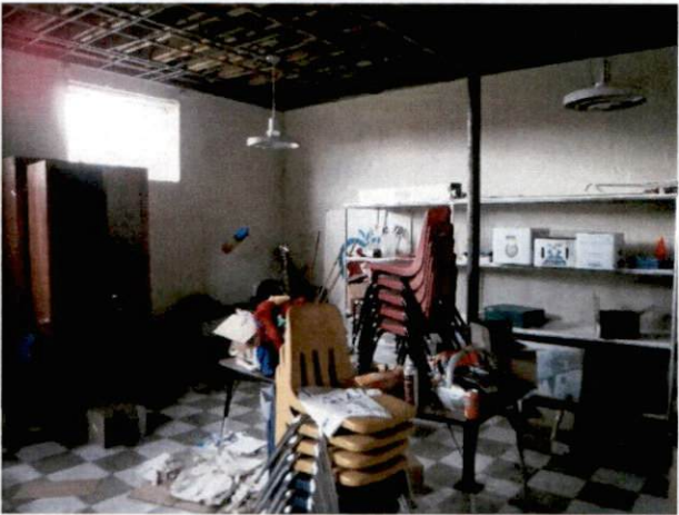
Photo #4 View of northeast storage room.
