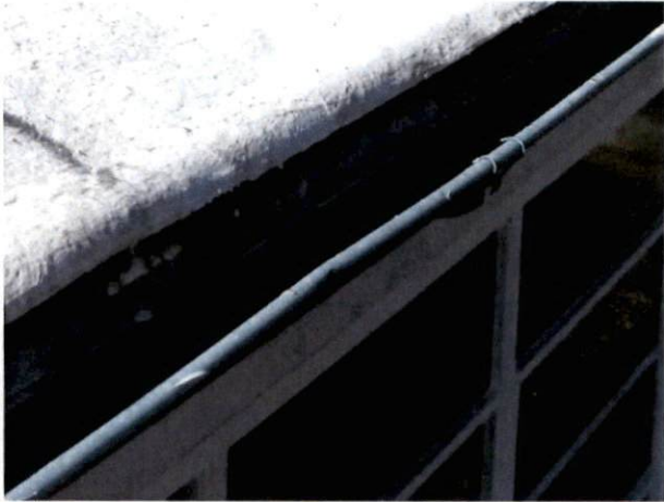
Photo #31 View of HA 27, non-asbestos containing black roof mastic on main roof.
