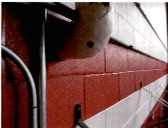
Photo #29 View of HA 25, non-asbestos containing hard TSI elbow with canvas wrap.
