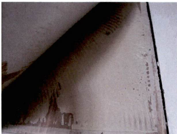
Photo #35 View of HA 30, non-asbestos containing beige FRP mastic.
