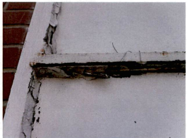
Photo #18 View of windows with HA 11, asbestos-containing white exterior window glazing.
