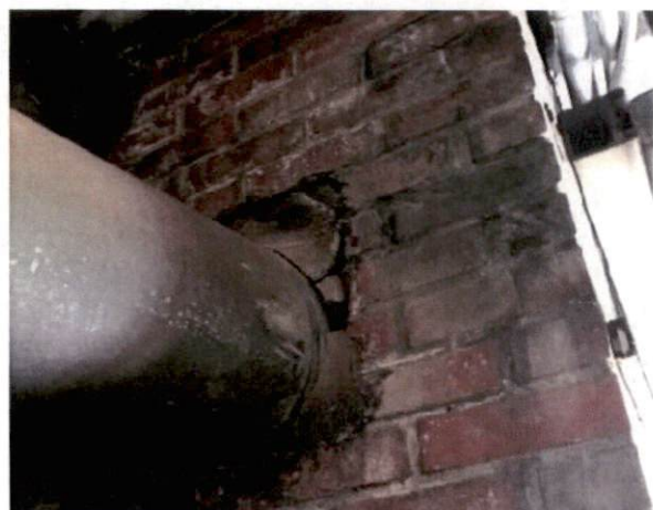
Photo #23 View of HA 17, non-asbestos containing concrete at flue.
