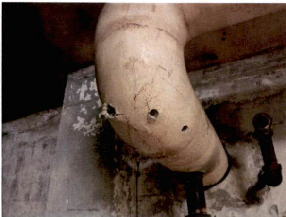
Photo #29 View of HA 25, non-asbestos containing hard TSI elbow.
