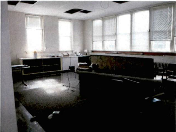
Photo #4 View of classroom.
