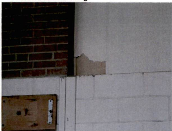
Photo #27 View of HA 23, non-asbestos containing beige FRP adhesive.
