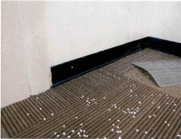
Photo #19 View of HA 15, non-asbestos containing 4" blue cove base and mastic.
