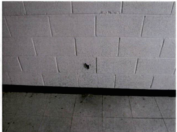
Photo #16 View of HA 9, non-asbestos containing 4" black cove base and mastic.
