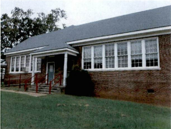
Photo #1 View of the front exterior.
