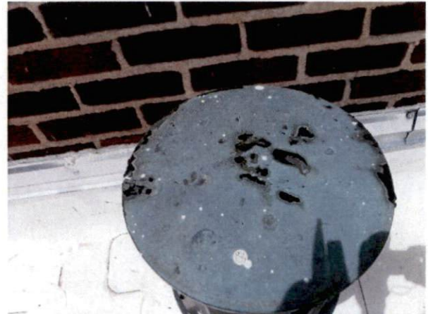
Photo #10 View of HA 4, non-asbestos containing black roof mastic on east roof.
