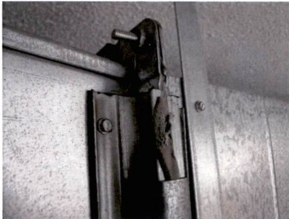
Photo #19 View of HA 13, non-asbestos containing gray HVAC duct putty.
