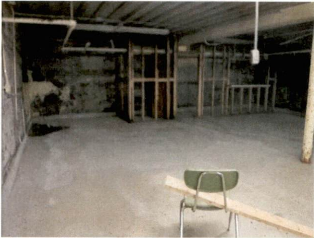
Photo #2 View of a basement.
