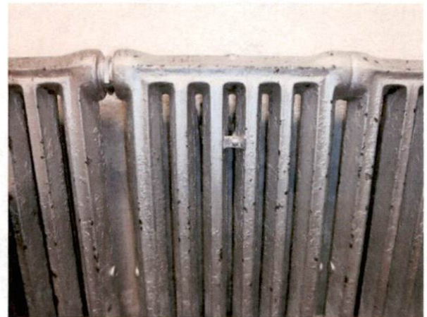
Photo #10 View of HA 5, non-asbestos containing silver paint on radiators.
