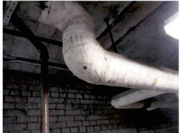
Photo #8 View of HA 2, non-asbestos containing hard TSI joint with tan canvas wrap.
