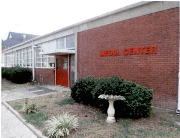
Photo #1 View of building exterior.
