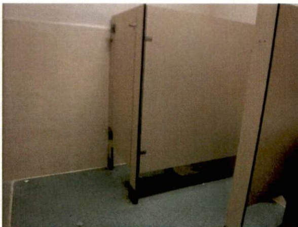
Photo #5 View of restroom.
