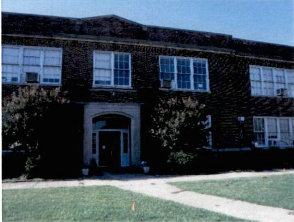
Photo #1 View of the front exterior.
