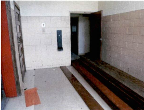
Photo #3 View of south entry.
