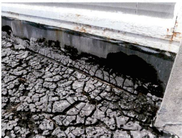
Photo #17 View of HA 11, non-asbestos containing black roof mastic on canopy.
