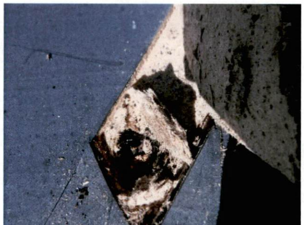
Photo #36 View of HA 32, non-asbestos containing built-up roofing on canopy.
