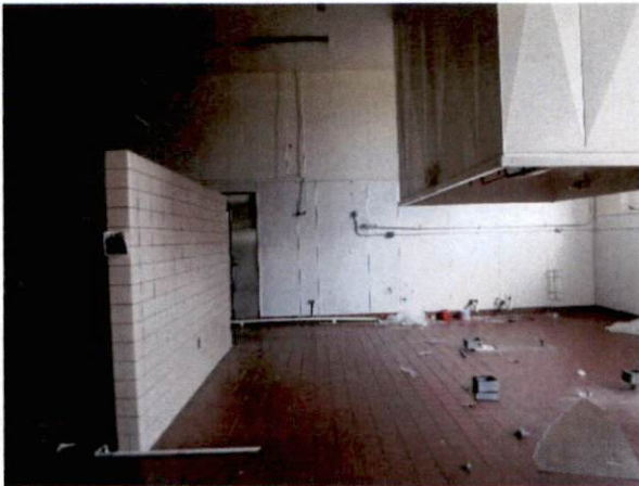
Photo #7 View of kitchen.
