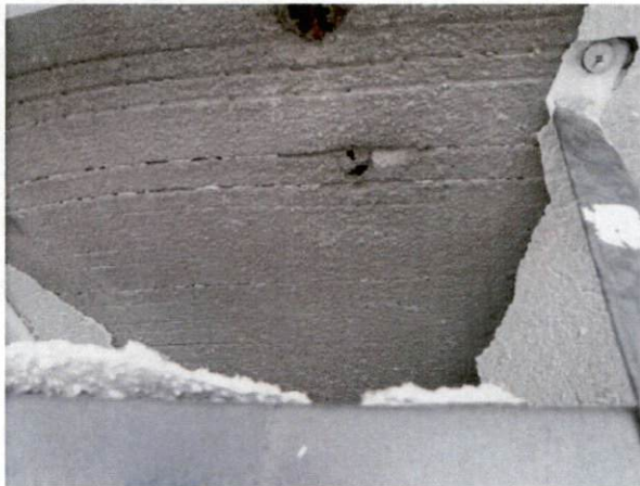
Photo #13 View of HA 6, non-asbestos containing textured ceiling plaster.
