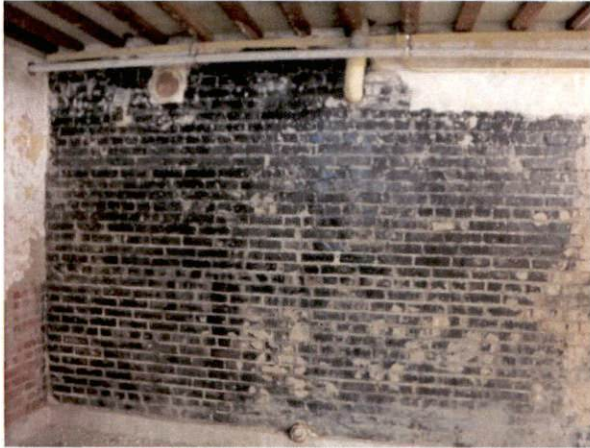
Photo #19 View of HA 11, non-asbestos containing black waterproofing.
